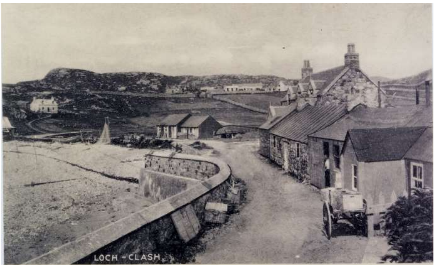
Loch Clash Shore—Early 20th Century Note addition of Pier House—2 storey stone building still standing
