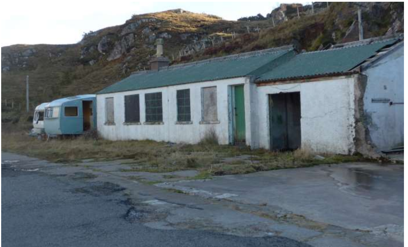
Loch Clash Pier—2016 Office Building—prior to demolition
